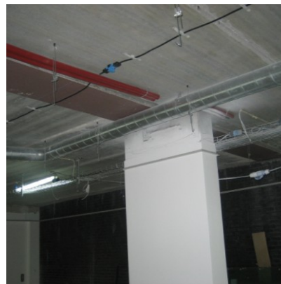
Figure 80 – Actual HVAC installation
