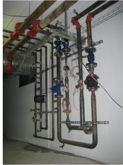
Figure 77 – Solved issue of MEP installations
