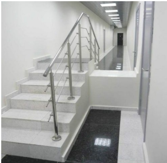
Figure 4 – Outcome of poor constructability analysis
