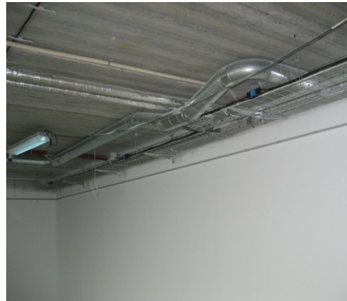
Figure 81 – Actual MEP and HVAC installation
