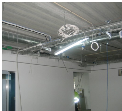
Figure 83 – Cable tray installation
