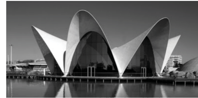
Concrete shell by Felix candela - thickness 30 mm!
