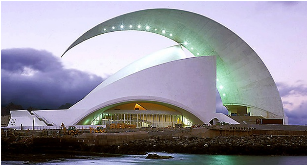
Figure 1.1: Auditorio de Tenerife, Canary Islands, Spain - Santiago Calatrava.[21].
